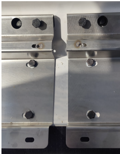
Figure 3.15, left: Bolts used for attaching anchor construction to the glass fibre construction.
