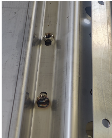
Figure 3.15, left: Bolts used for attaching anchor construction to the glass fibre construction.
